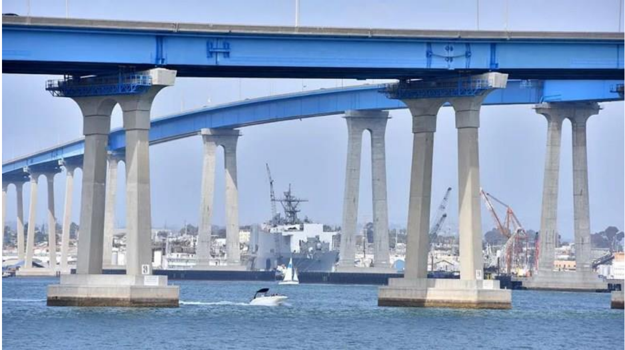
The San Diego-Coronado Bridge has seen over 450 suicides over the years. Photo by Chris Stone
